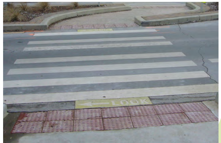
Mid-block crossing with a marked crosswalk and “z” pattern island refuge
