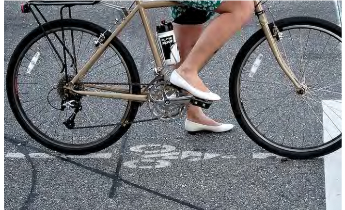
Bicycle detection loop in the pavement and marked with a bicycle detector symbol
