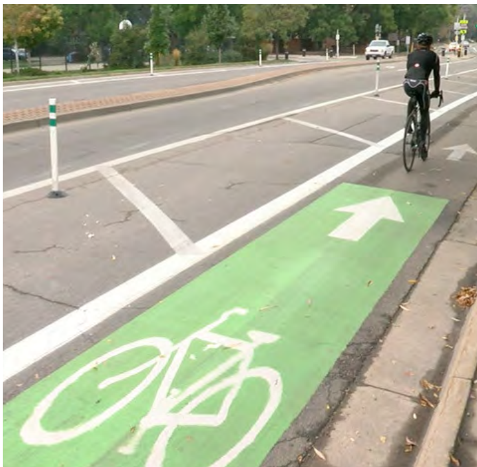
Green color pavement in separated bicycle lane
