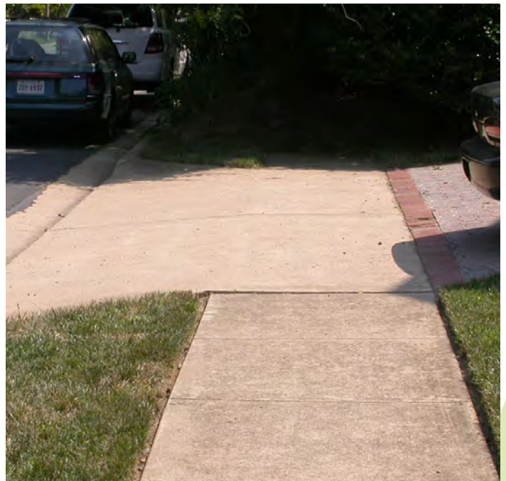
Continuous sidewalk material across driveway vehicular path.
