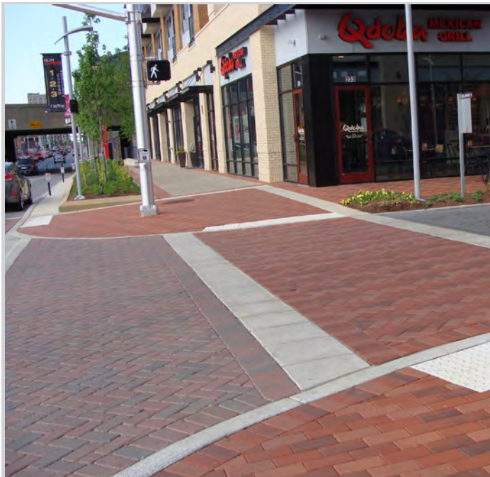
Flush crossing with textured vehicular ramps and color contrast between vehicular and pedestrian zones
