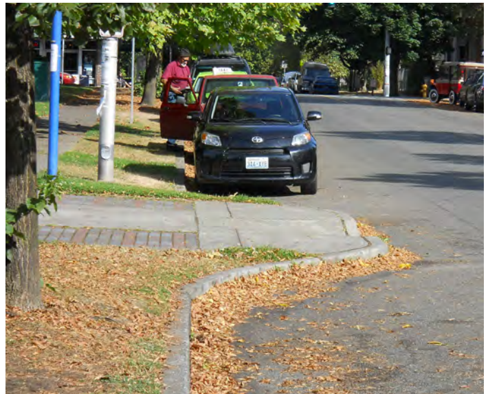
Bulbouts at intersections or mid-block help shorten pedestrian crossings and visually narrow the roadway
