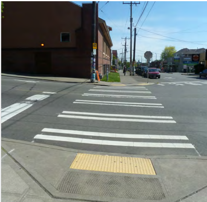
Standard painted crosswalk with ADA compliant curb ramps
