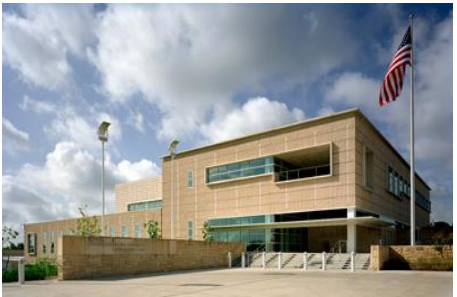
Figure 5 – CTECC is an excellent example of state, county and municipal cooperation that has led to improved TIM in the CAMPO Region.
