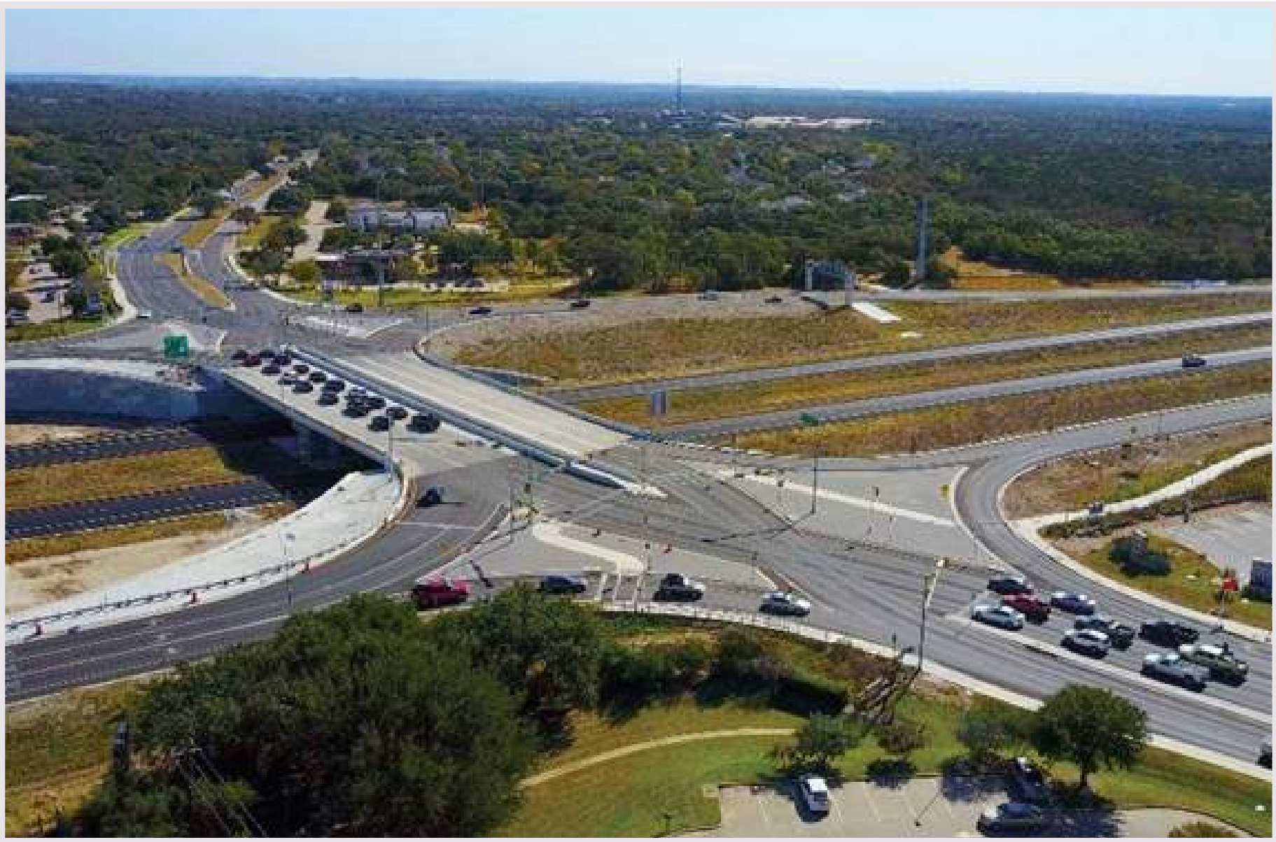
DIVERGING DIAMOND INTERCHANGE (DDI)
