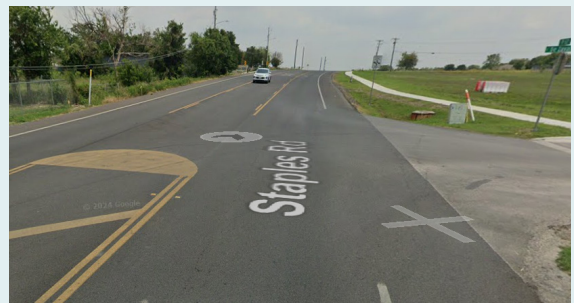
FM 621 After. Source: Google Street View.
